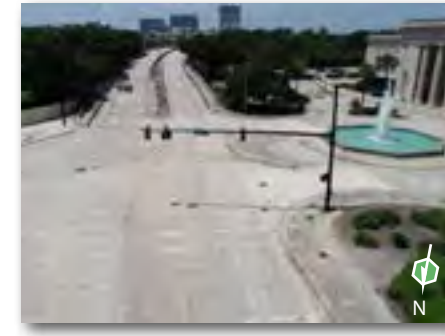
Existing conditions on the Park Street Viaduct
