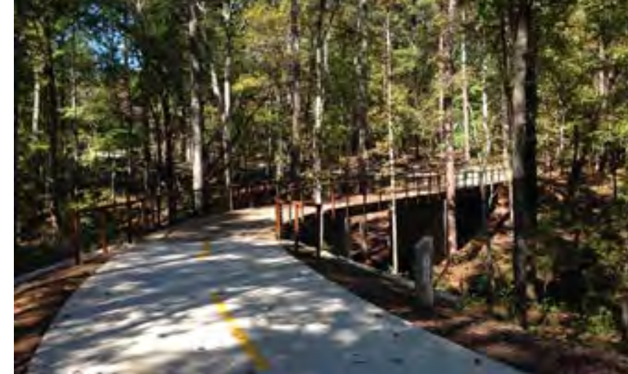
Custom steel bridge allows the trail to naturally blend into wooded areas.
