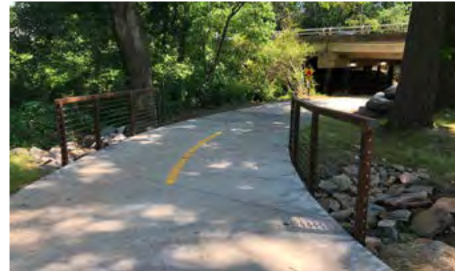
An example of the cable handrail with cor-ten steel posts and top rail.
