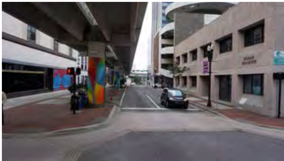
Opportunities to activate the vacant buildings in Downtown Jacksonville by building the proposed trail segment through this area.
