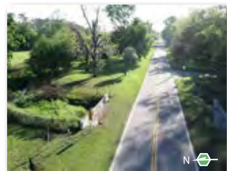
Existing conditions on McCoys Creek Boulevard looking east
