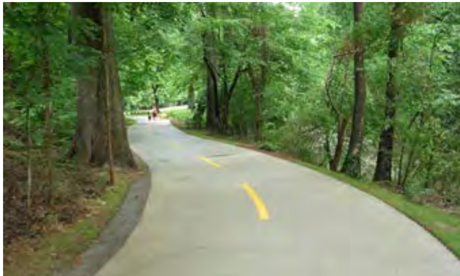
An example of incorporating the pervious concrete strip along the trail edge
