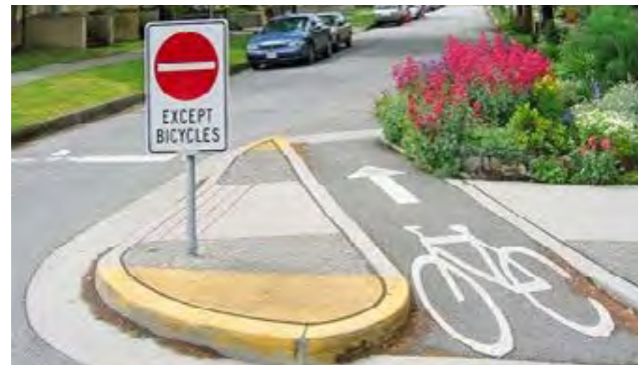
Neighborhood Greenway example showing limited vehicle entry while utilizing signage and pavement markings for cyclists.
