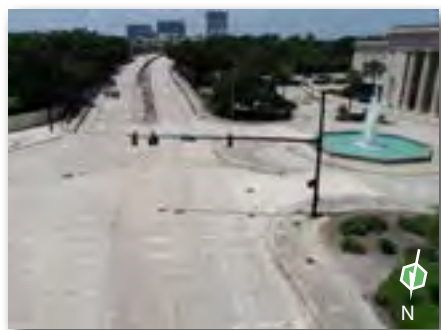
Existing conditions on the Park Street Viaduct
