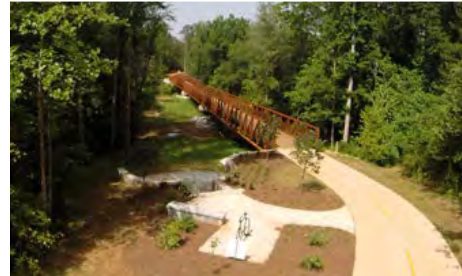
Prefabricated steel bridge allows the trail to cross above existing roads and waterways.
