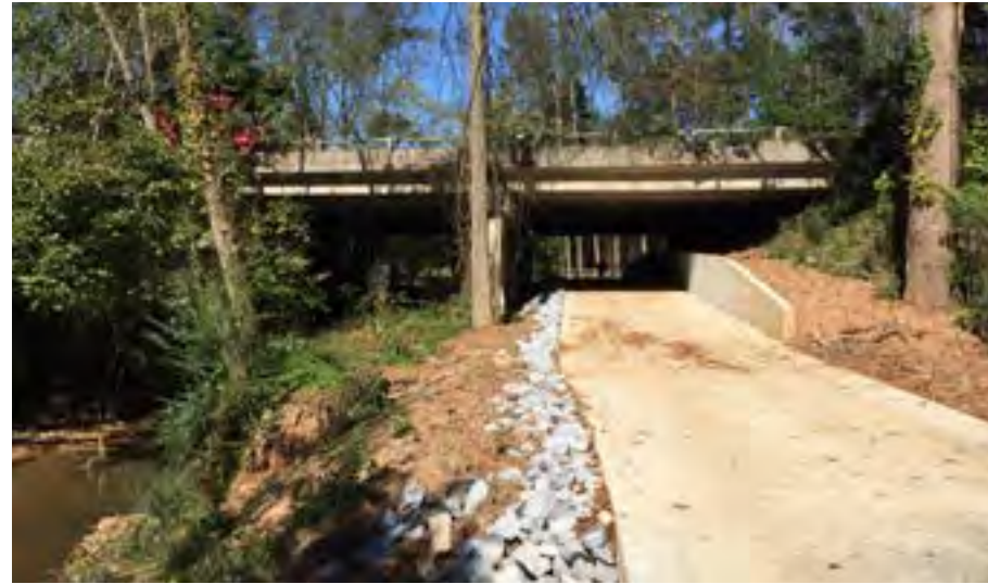
Multi-use trail going under a roadway
