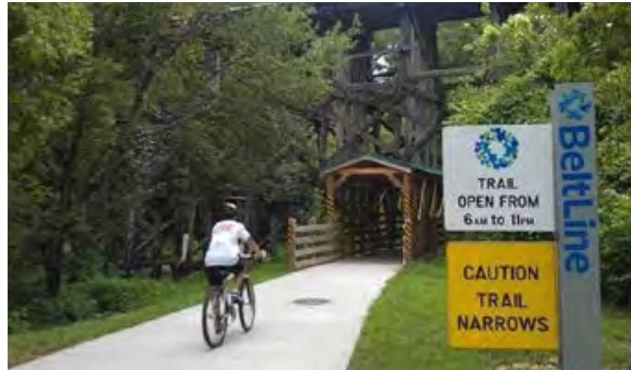
A canopy protective structure over the trail is required when going beneath railroads
