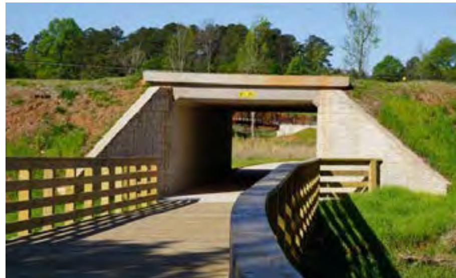
Box culvert structure allows the trail to pass under a roadway
