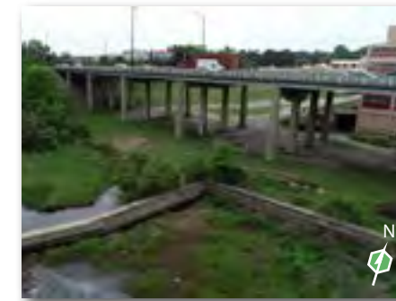
Existing conditions at south of Arlington Expy
